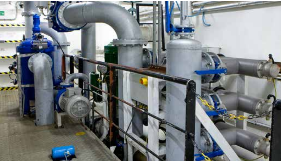
Optimarin System installed onboard
