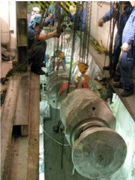
Rigging replacement shaft into engine room via hole cut in passageway floor
