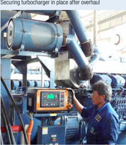
Test running/commissioning of engine
