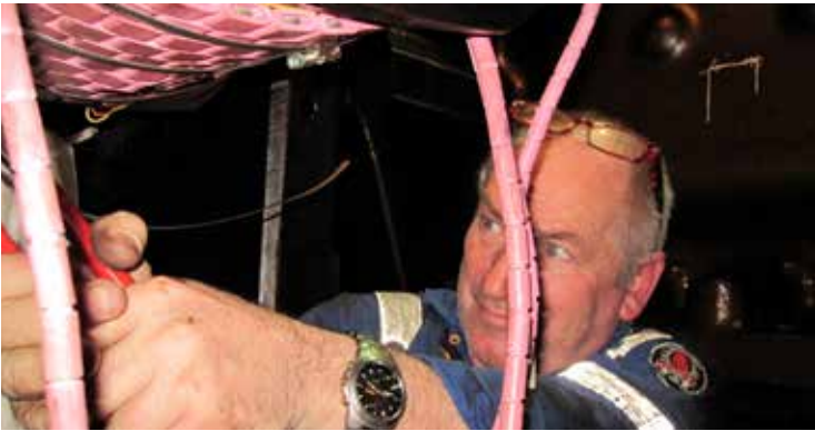
Installation of ceramic tile heating blankets for annealing
