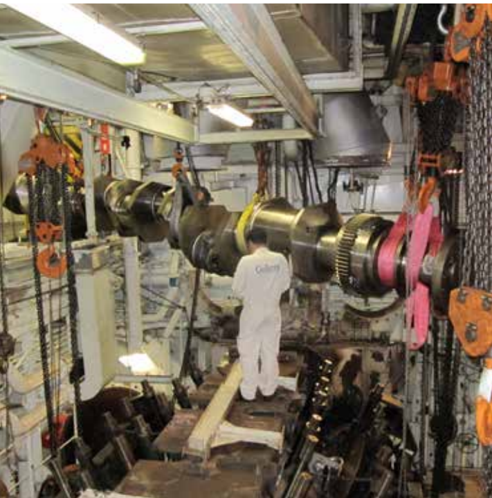
Rigging of condemned crankshaft from the engine room
