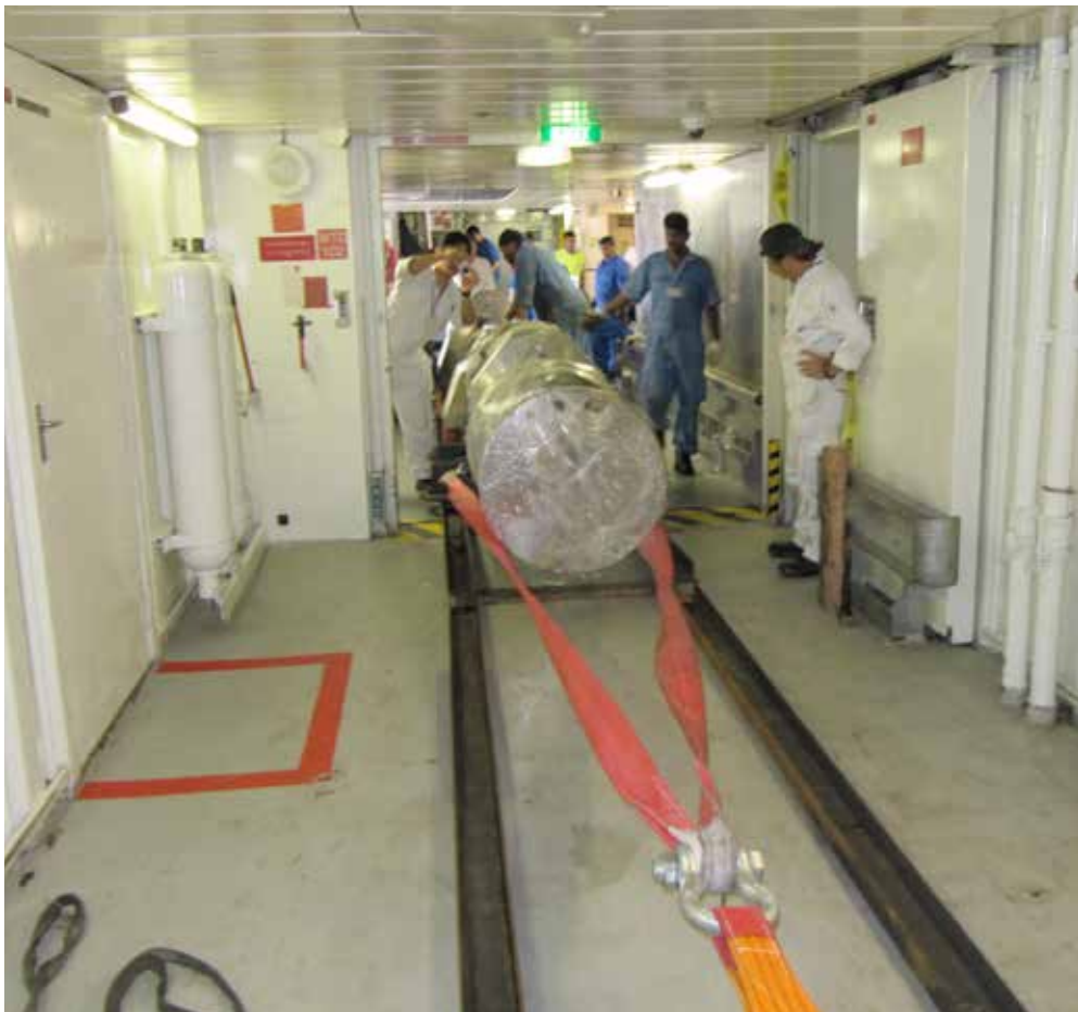
Transfer of replacement crankshaft down 80 meter passageway
