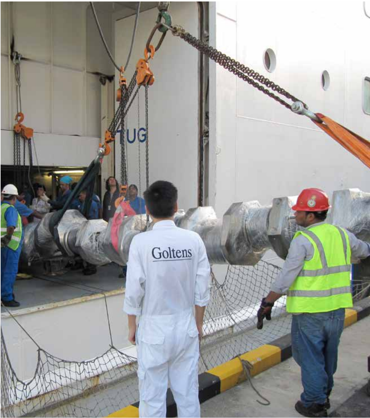
Rigging of replacement crankshaft onboard during port call in Singapore
