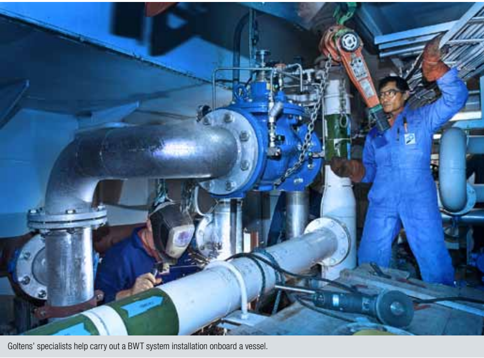
Goltens' specialists help carry out a BWT system installation onboard a vessel.
