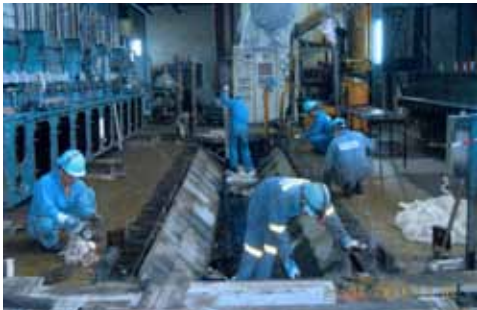
Modification of the concrete foundation
