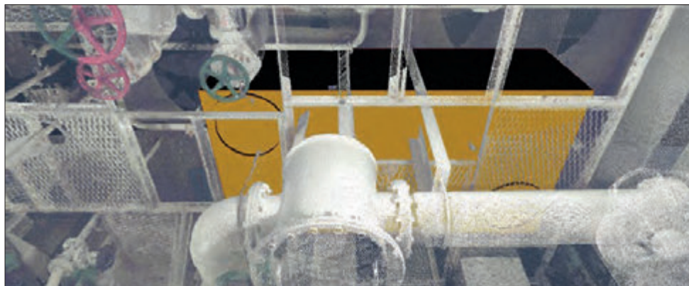
Thermal oil drain tank.
