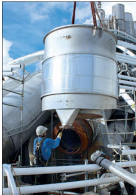
Rigging exhaust gas scrubber section aboard.
