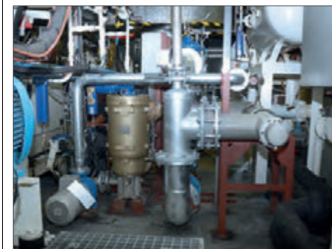
BWT system section installed on board PGS Apollo.
