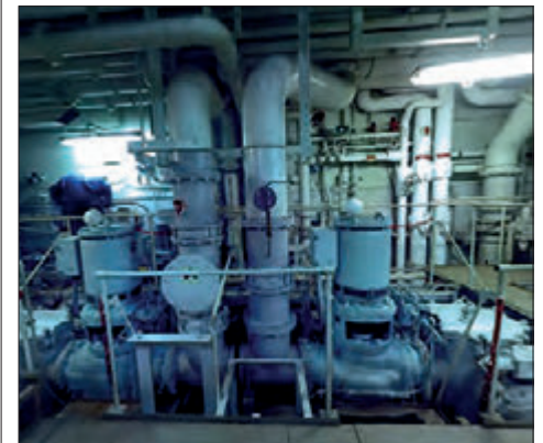
Existing ballast pump area (pre-installation).
