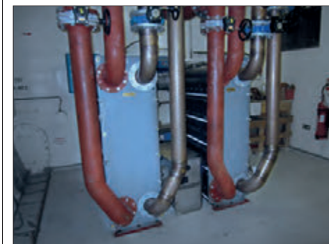
Part of the main engine cooling system installed on board.
