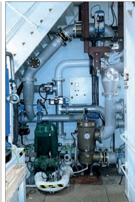
Hyde Guardian Gold 300m 3 /hour system installed on board Polar Queen.
