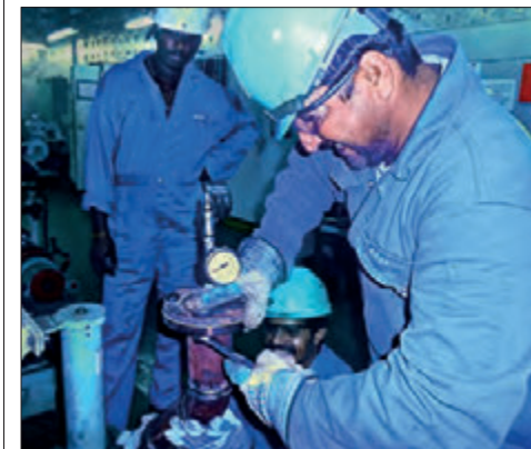
Preparing for fuel system pressure testing.
