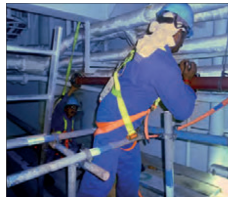
Installation of fuel transfer line on board.
