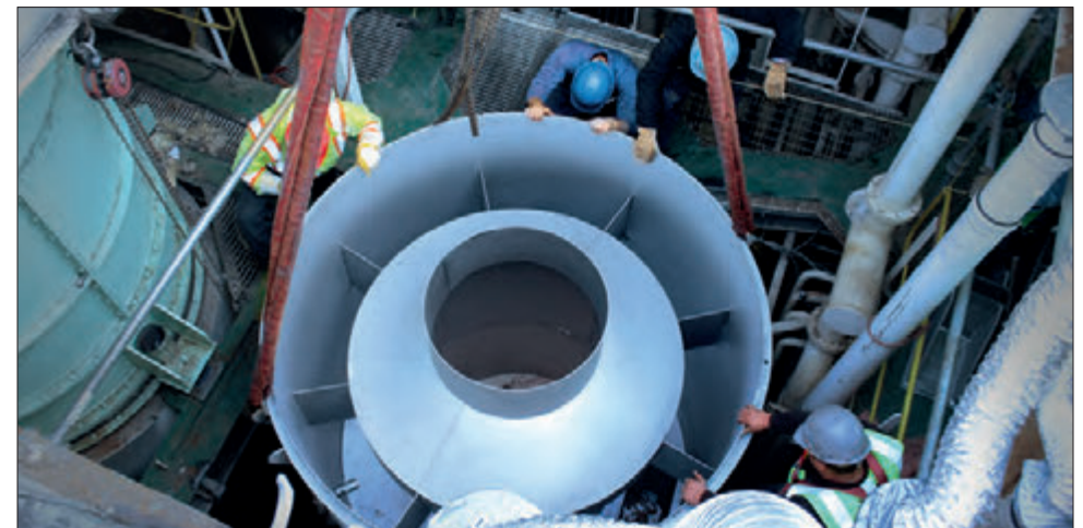
Rigging scrubber section into the ship.
