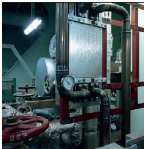
LSGO Cooler installed on board.
