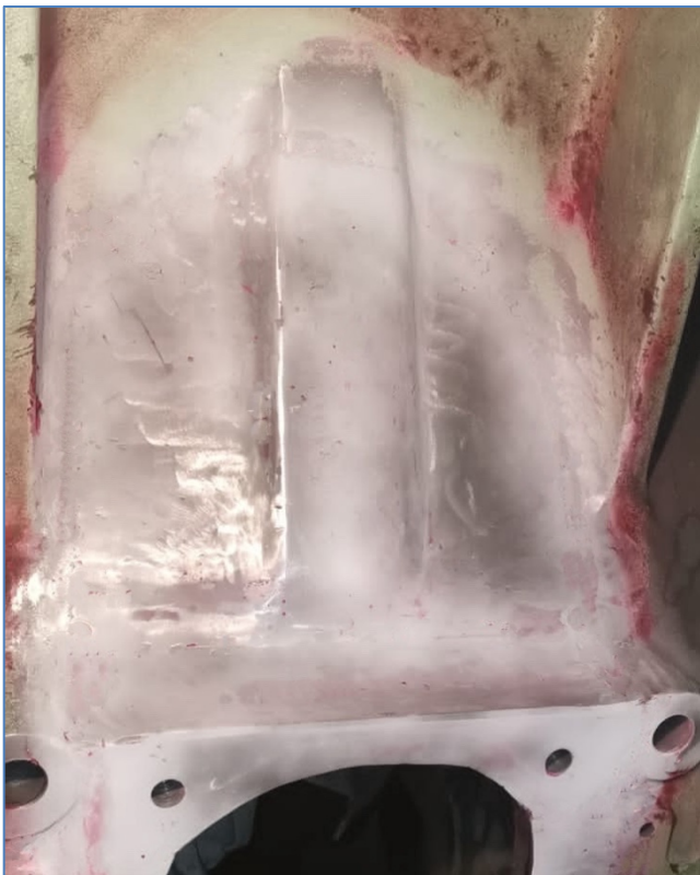
Figure 4: Die penetrant crack test of repaired surfaces
