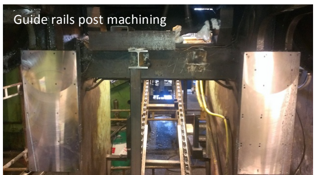
XY Milling of guide rails in progress
