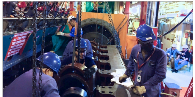
Replacement of bearing caps to check line bore
