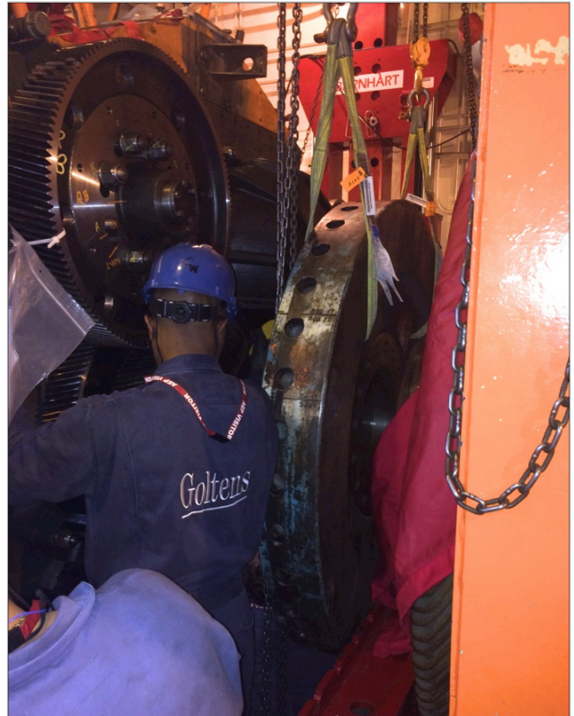
Rigging flywheel into position
