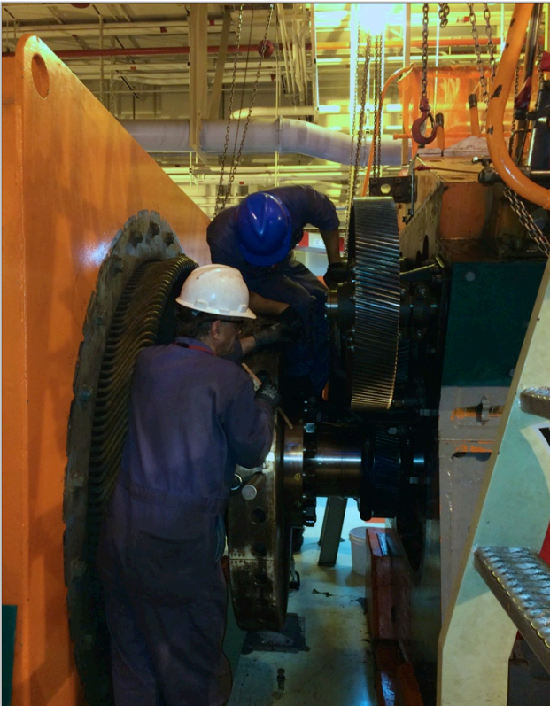
Reassembly of front end of the engine
