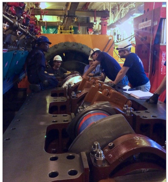
Replacement of bearing caps to check line bore
