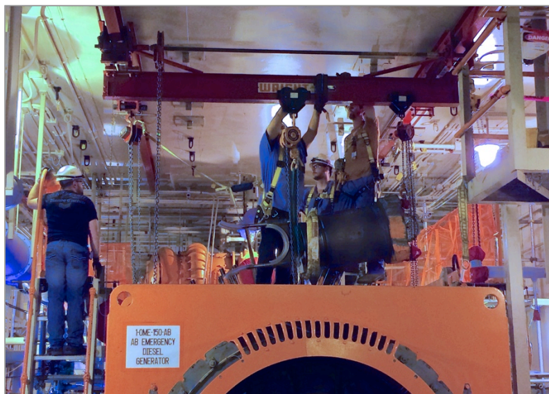
Rigging power pack into place during rebuild
