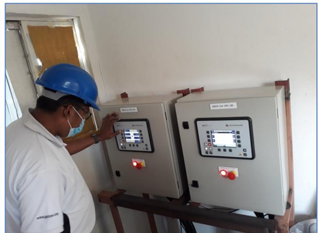
Figure 3: Configuration of Woodward easYgen controllers
