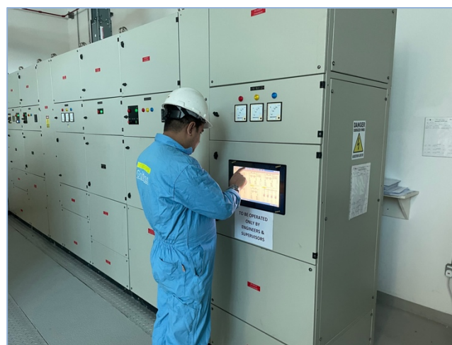
Goltens' ECS technician performing setup of HMI after installation
