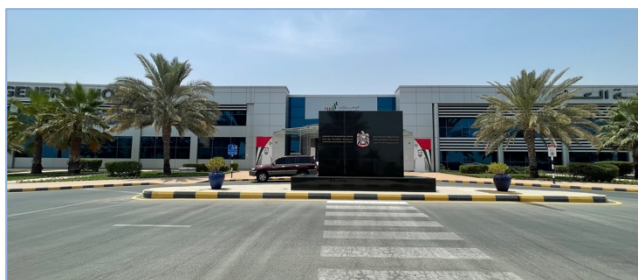
UAE Hospital where upgrades were completed
