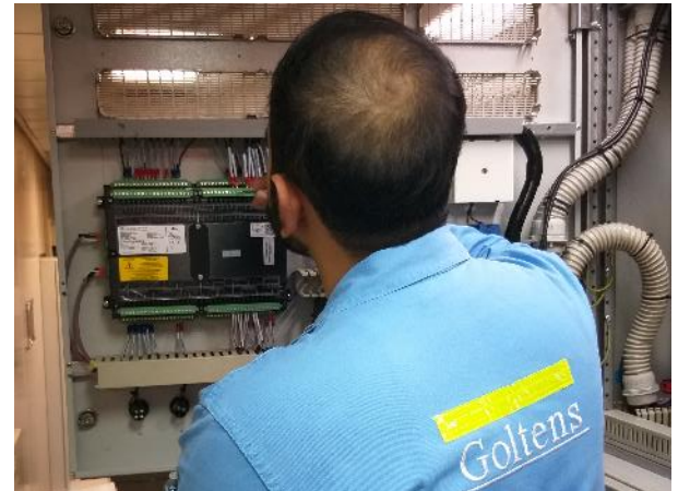
Figure 2: Technician installing new easYgen
