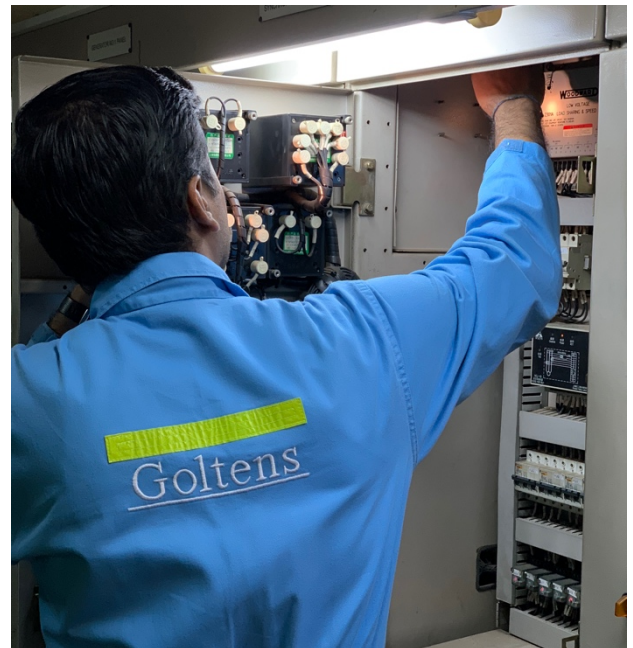
Figure 2: Removal of the Analogue Woodward 2301A LSSC
