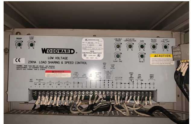
Figure 1: Legacy Analogue Woodward 2301A LSSC
