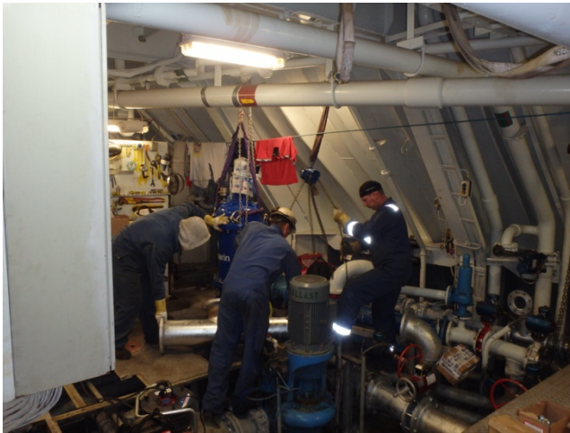
Figure 4: Goltens' team rigging piping into place
