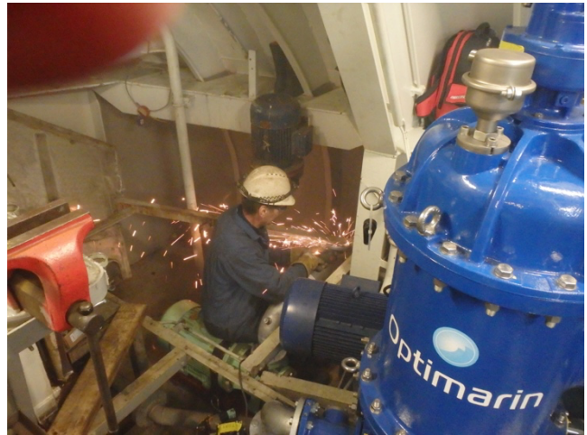
Figure 5: Making required adjustments to deck plate supports
