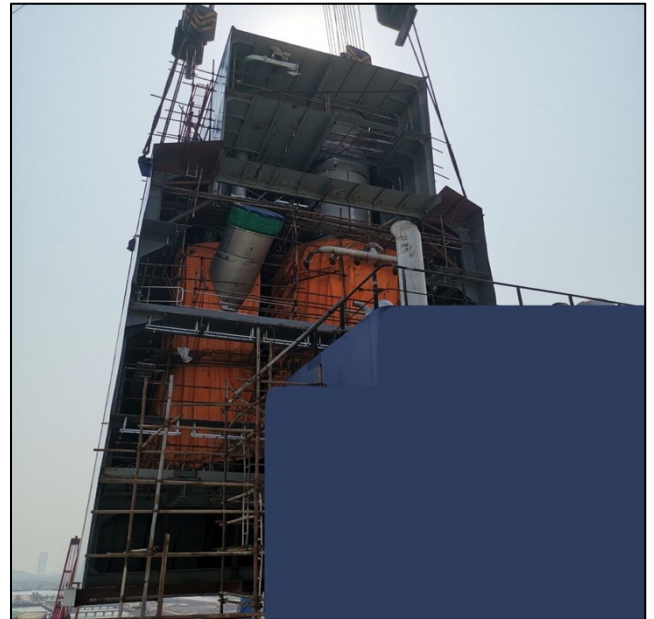
Figure 1: New Scrubber casing integration
