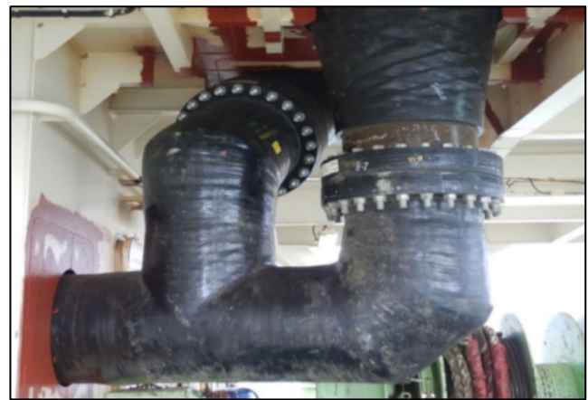
Figure 9: GRE Scrubber Discharge Line installed
