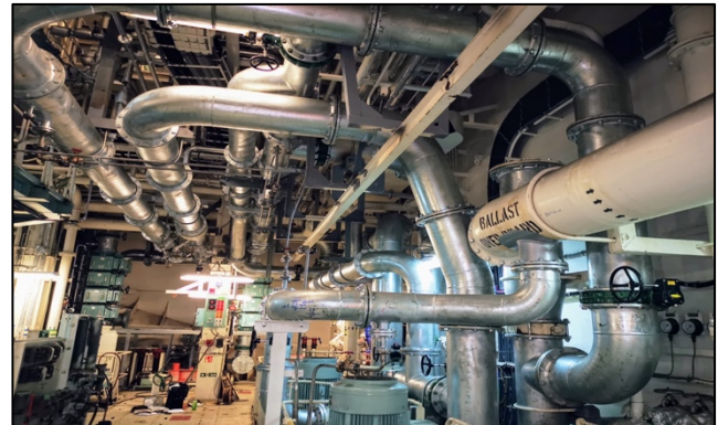
Figure 7: BWTS Unit installed in Engine Room
