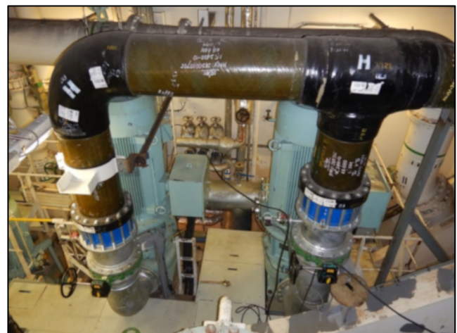
Figure 11: SW pumps for Scrubber Feeder Line installed
