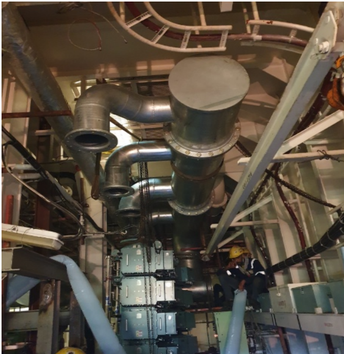
Figure 9: Installation of Big Bore Spools with ECUs
