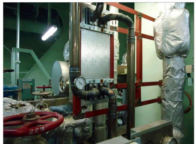
LSGO Cooler installed onboard
