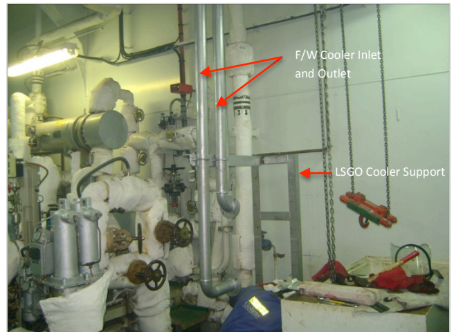
Installation of fresh water piping and cooler support
