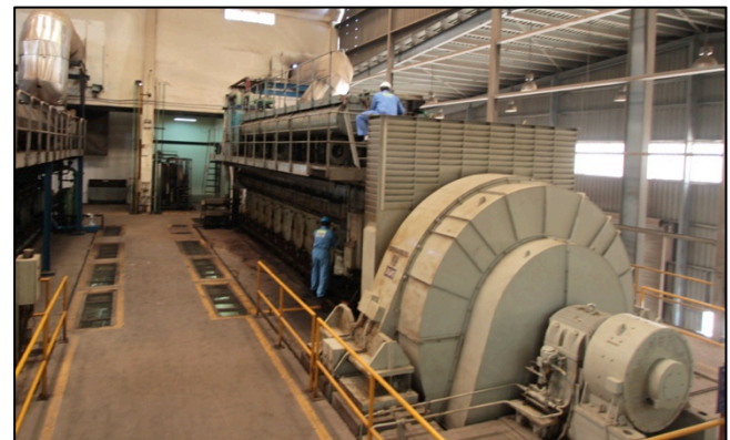
Goltens Diesel Technicians finalize work on one of the MAN B&W 9L58/64 engines at Star Cement
