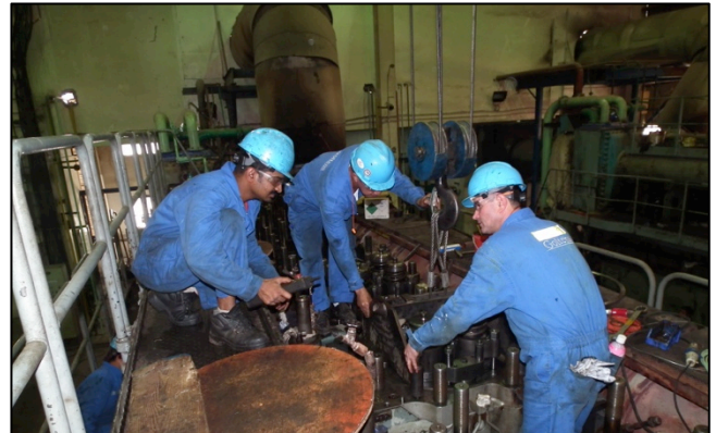
Goltens' Diesel Technicians fastening the lifting yoke to remove a cylinder head from the engine
