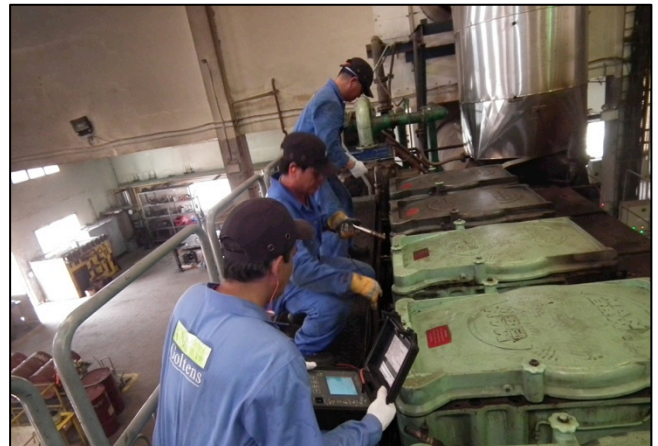
Goltens technicians performing operational performance tests ahead of overhaul
