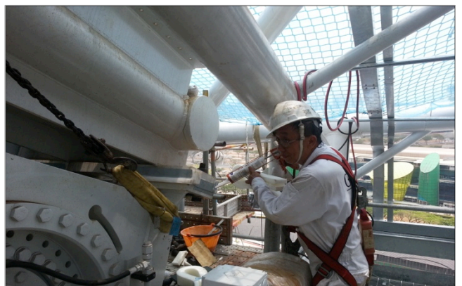
Filling in gaps on the winch footings
