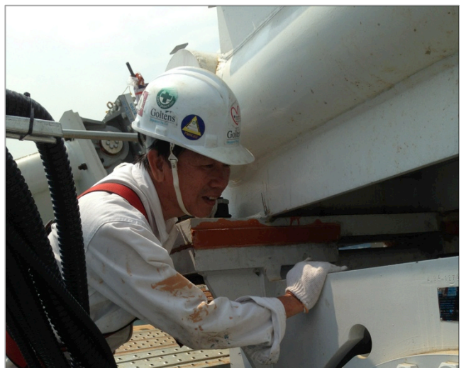
Specialist performs final inspection of foundation
