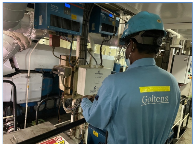
Figure 2: Goltens’ Controls Engineer installing the Smart Box to work with the new UG25+P3 installation
