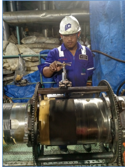
Figure 5: Machining shaft to nominal dia.
