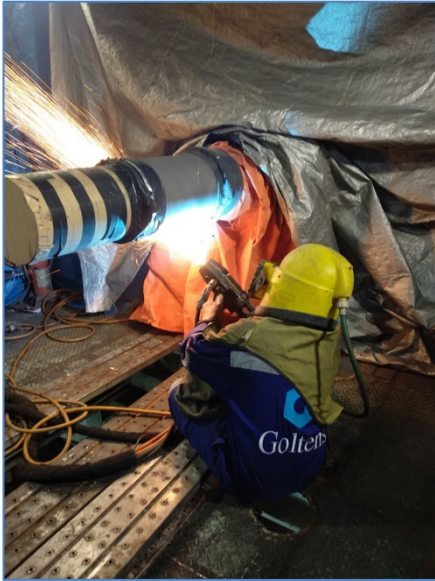
Figure 4: Thermal Spraying of agitator shaft
