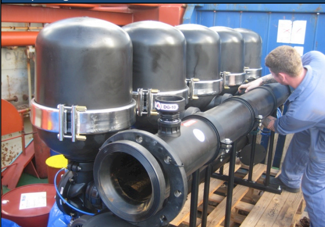
Preparing filter units for installation
