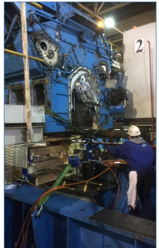
Lowering block back to bedplate
