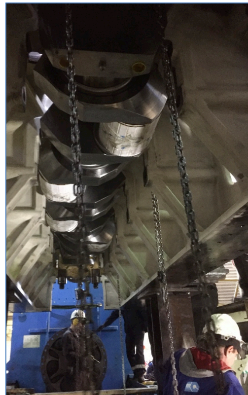
New crankshaft lifted into position
