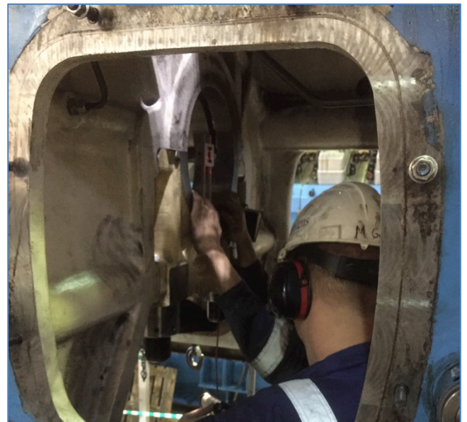
Laser alignment check of main bearing pockets
