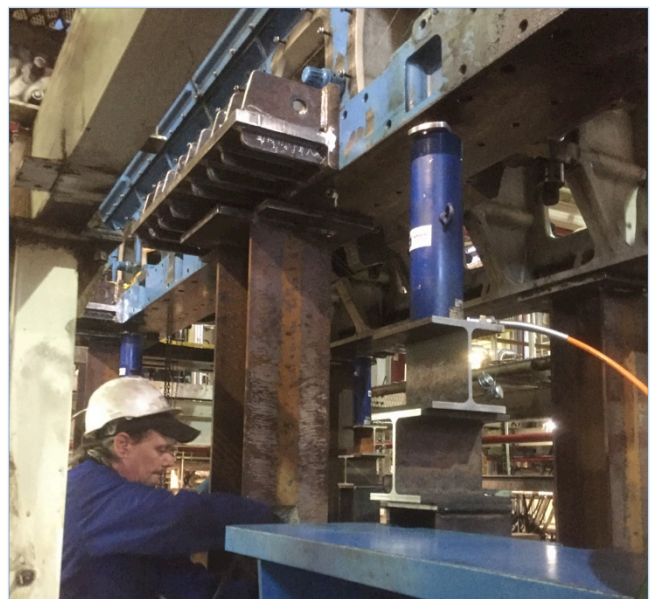
Block lifted with vertical steel supports installed
