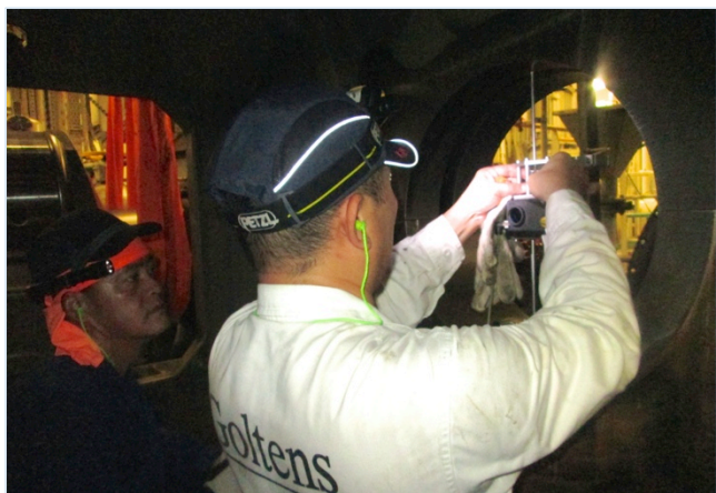
Laser check of main bearing pockets
