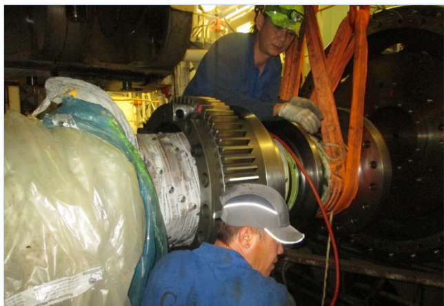
Rigging crankshaft into position
