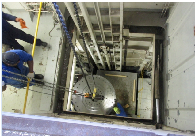
Rigging of new flywheel into engine room
