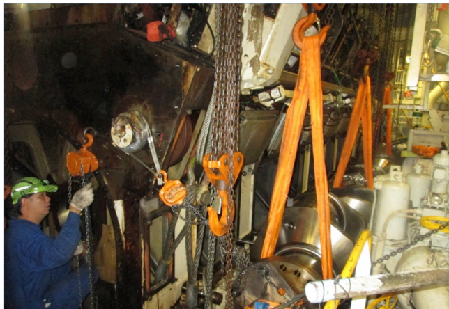
Rigging of condemned crankshaft from engine
