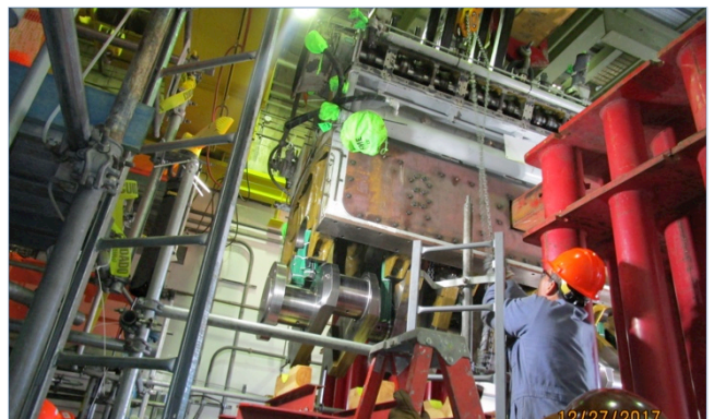
Lowering crankshaft onto skid for removal
