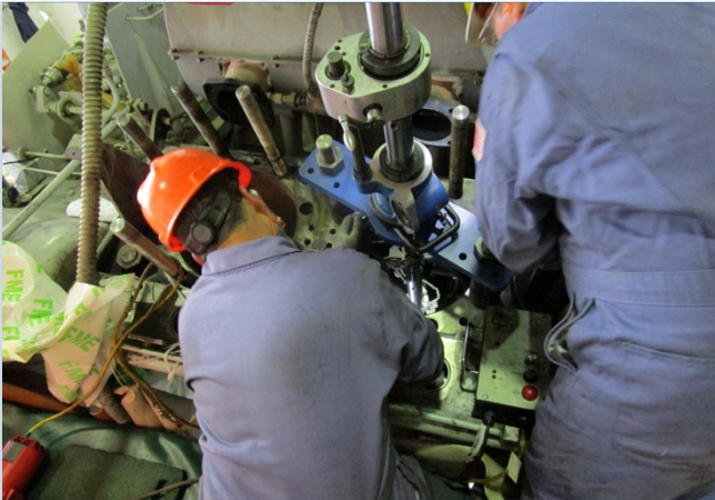
Boring lower liner landing after metal stitching
