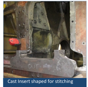
Damaged section removed
