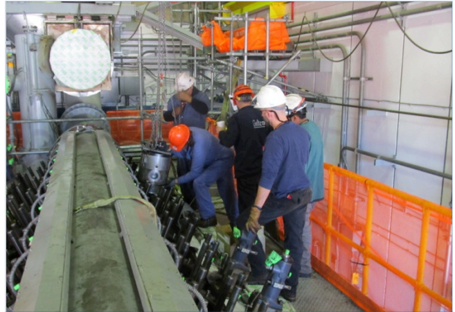
Reinstallation of power packs
