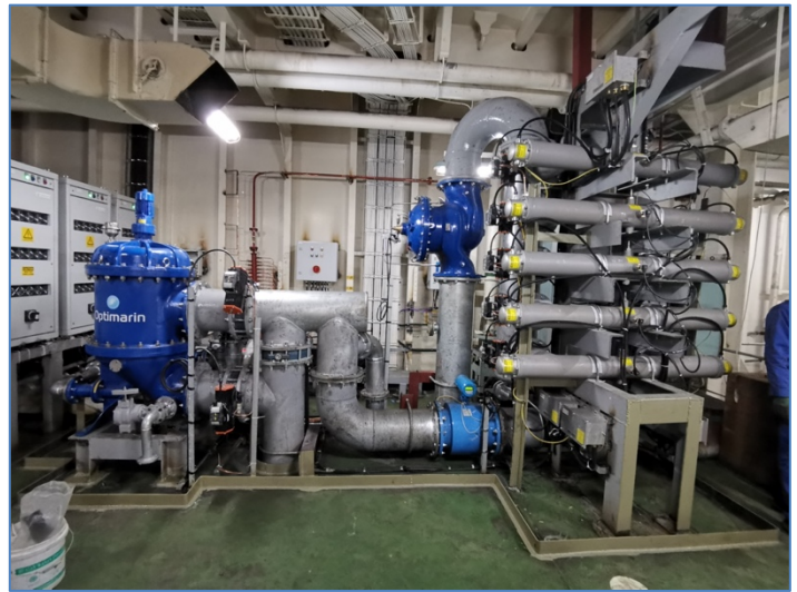
Figure 5: Main components of Optimarin system installed per design
