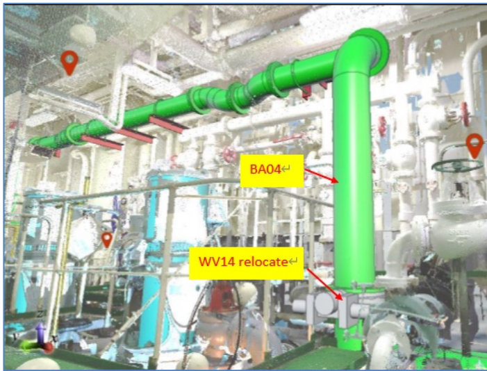
Figure 10: 3D Model of tie in required to existing pipe spool
