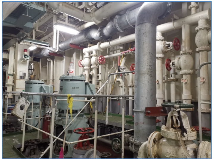
Figure 11: Spool tie in completed
