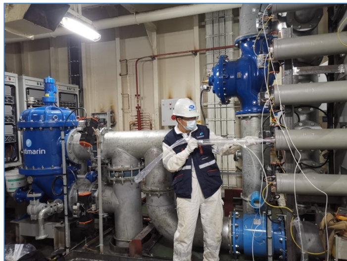
Figure 12: Commissioning – Insertion of UV tube
