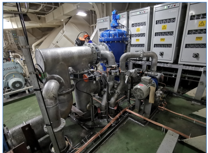
Figure 9: Filter and back flush pump installed
