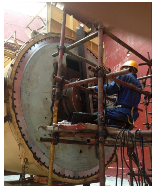
2.75 meter flange facing in progress
