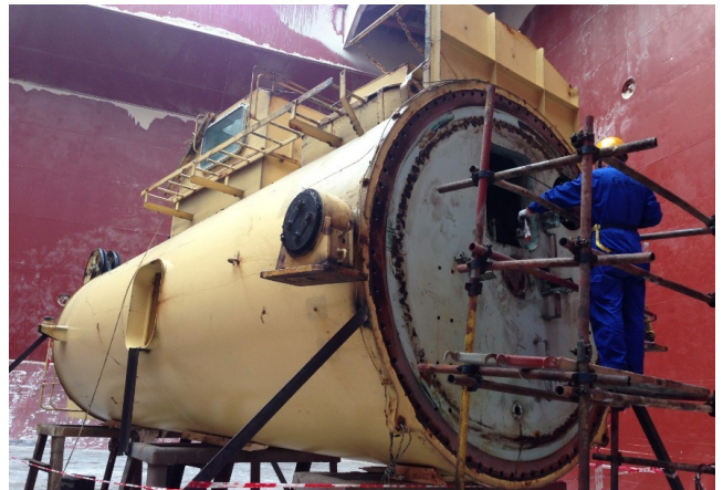
Inspection of damaged crane pedestal flange
