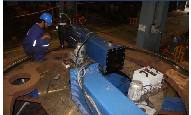
Machining of the 3.43 meter flange in process
