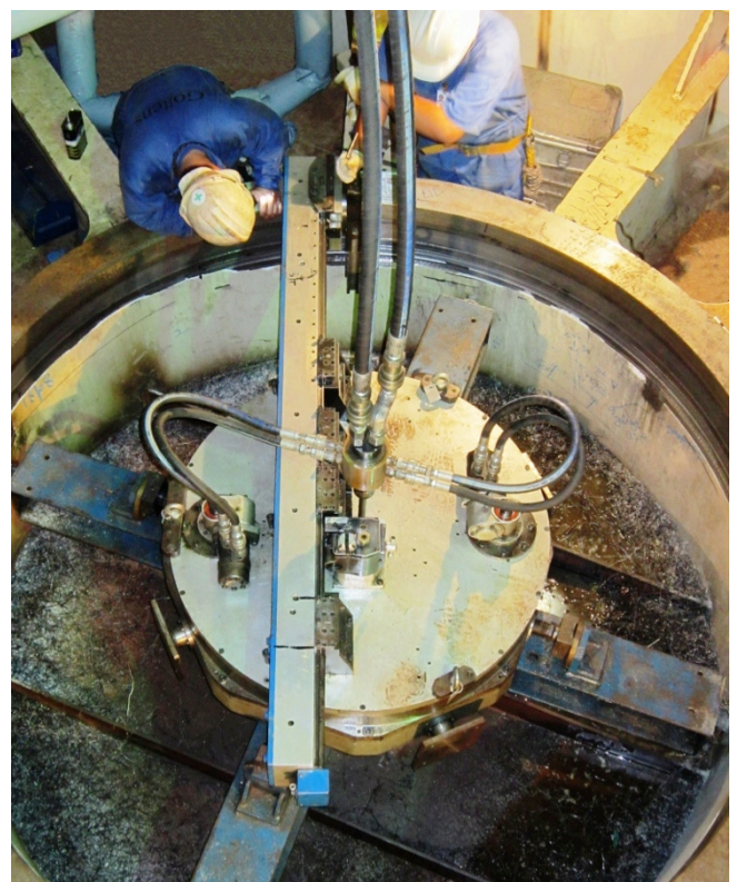
In-Situ machinists adjust flange facer during job
