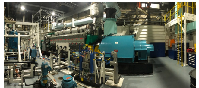
Figure 4: Replacement EDBG installed and operational
