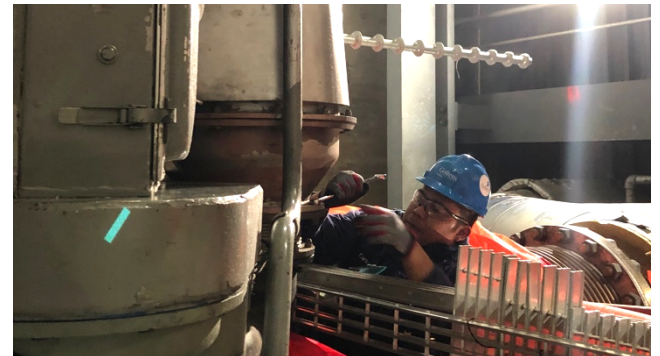
Figure 3: Installation of EDBG Exhaust Bellows
