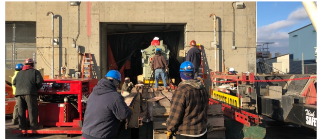
Figure 2: EDBG being slid into powerhouse on skid
