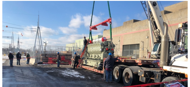
Figure 1: Rigging replacement EDBG from trailer to skid
