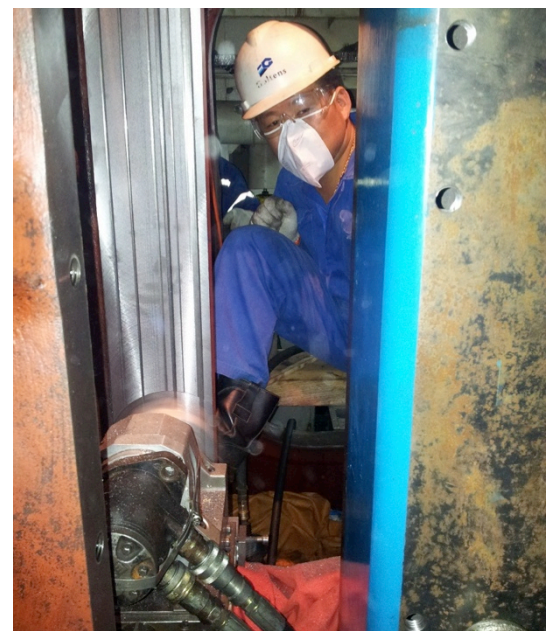
Milling in process on damaged guide rail
