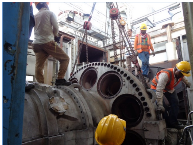
Figure 2: Removal of Turbine casing
