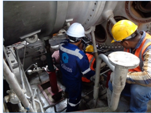
Figure 4-5: Dismantling turbine and accessories
