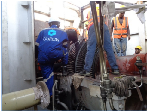
Figure 4-5: Dismantling turbine and accessories
