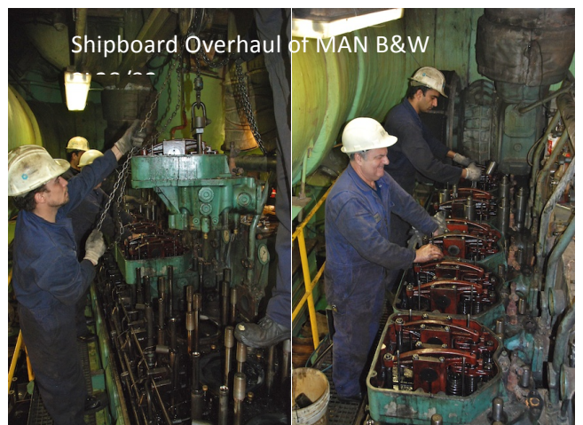
Retapping bolt holes and replacement of exhaust bellows
