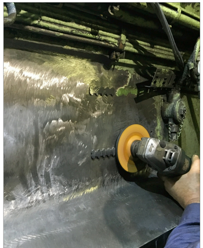
Finish grinding after locks were inserted
