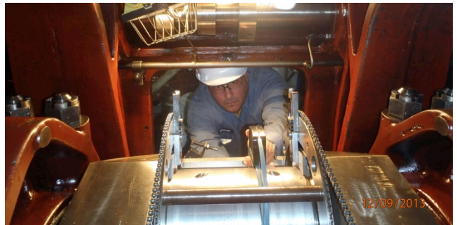
Checking the journal diameter during machining
