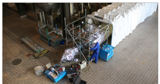
Machining of the damaged rotor shaft in progress
