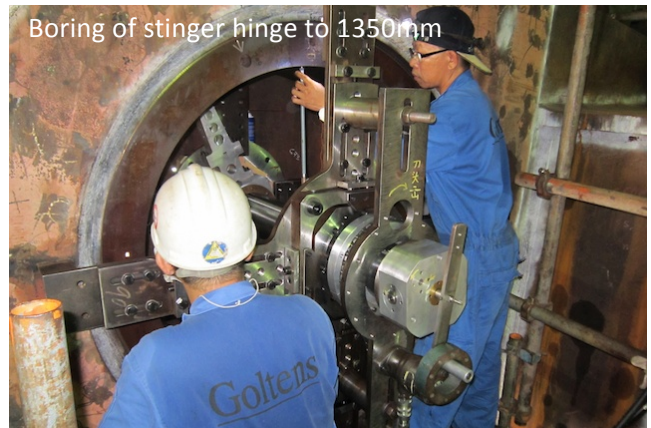
Checking diameter of the bore
