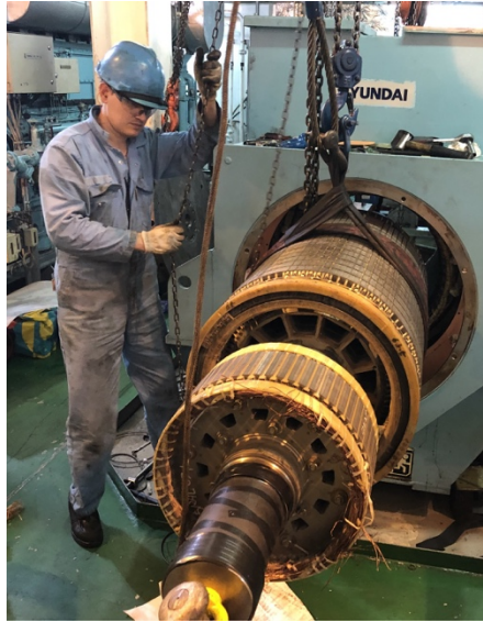
Figure 5: Rigging damaged alternator
