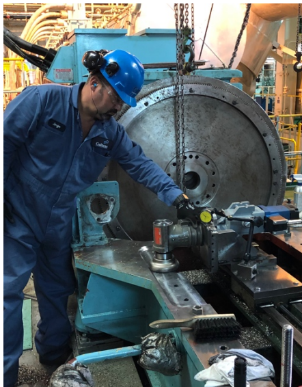
Figure 7: Finish milling recess in bedplate
