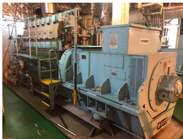
Figure 10: Engine rebuilt and returned to full service
