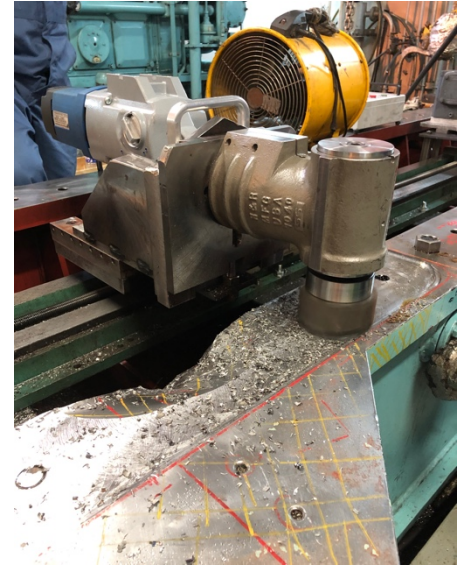
Figure 6: Milling damaged area
