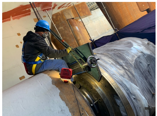
Figure 2: Installation of milling machine on prefabricated brackets
