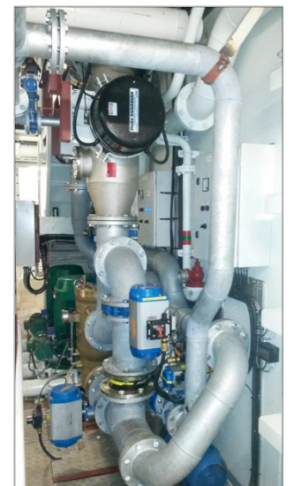
Hyde Guardian System installed onboard per design
