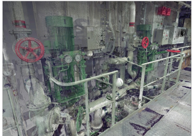
3D scan of Ballast Pump area – pre BWTS installation
