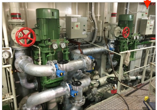
Hyde Guardian System installed per model/design
