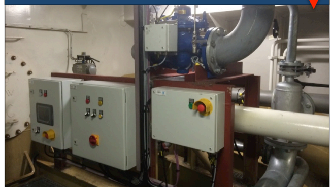
Control cabinets and control valve installed onboard
