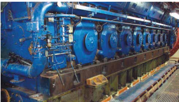
Chockfast® application on 150 ton Sulzer 16V ZAL 40 Main Engine
