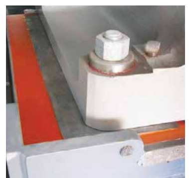
Chockfast® application on Motor Foundation
