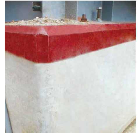
Single deep pour minimizes downtime, while Chockfast® effectively damp vibration
