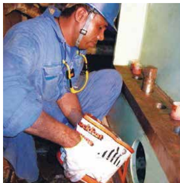
Chockfast® application on Main Engine
