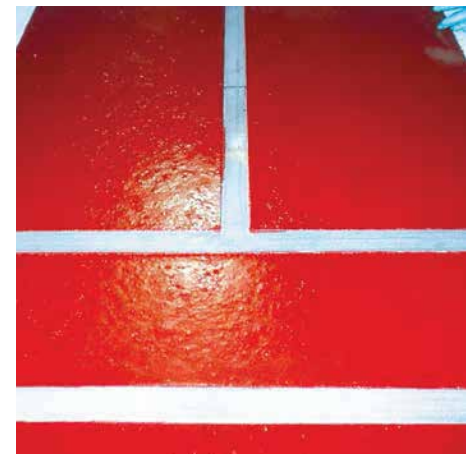
Skid module pre grouted with Chockfast®
