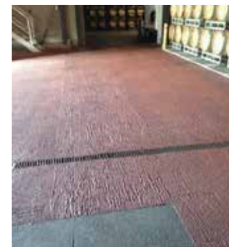
Entire factory floor coated with AST product
