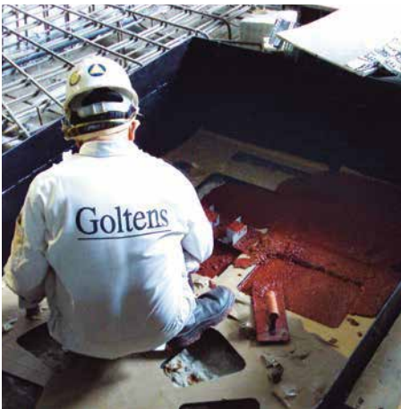
Surface preparation prior to grouting
