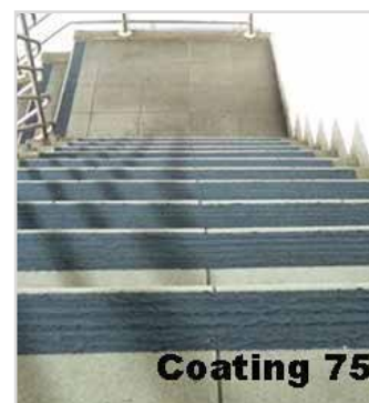
AST enhance the safety of the staircase
