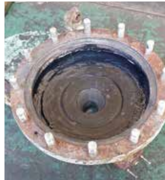
Devcon rubber application on pump cover
