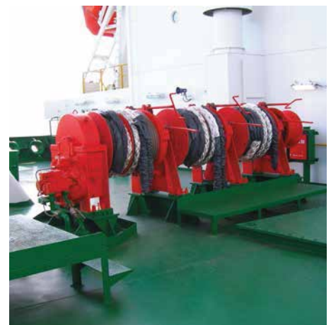
Chockfast® application on main deck machinery
