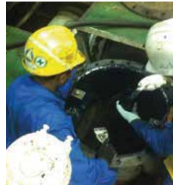
In situ repair on pipe
