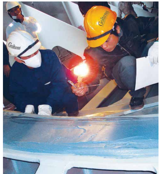
Specialists checking on the thickness of the Phillymastic prior to tank installation
