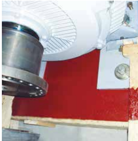
Re-grout of poorly aligned Pump, now on Chockfast®
