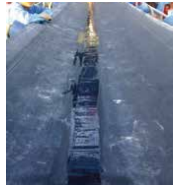
Conveyor belt repair
