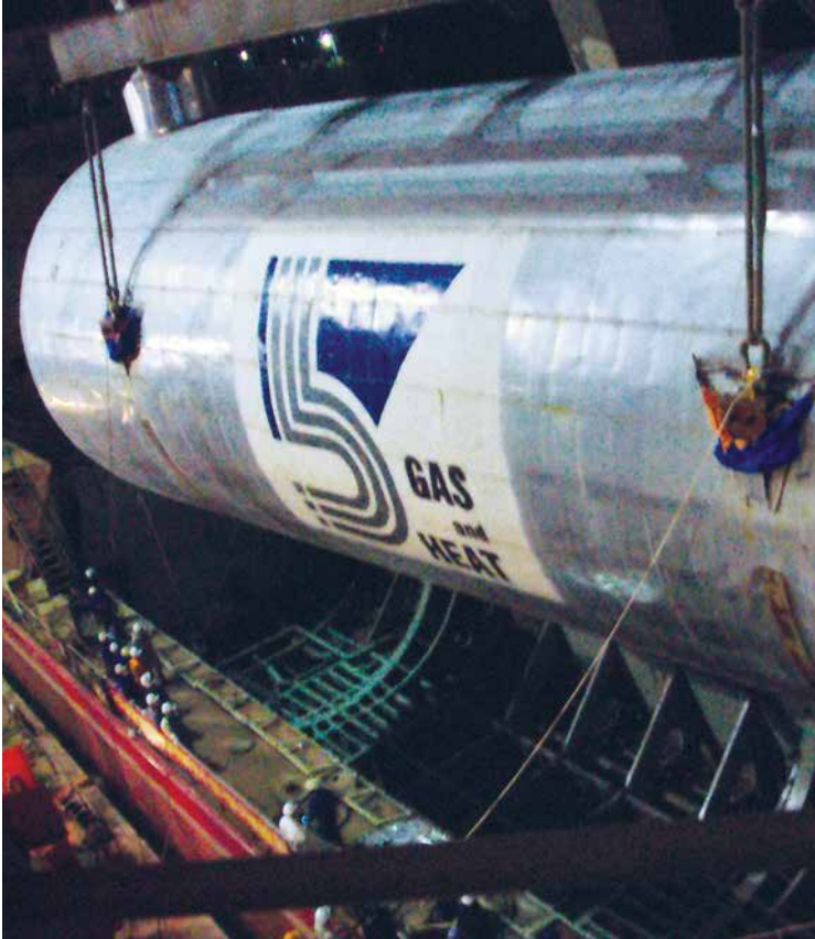
New Ethylene tank ready for Phillymastic installation onboard
