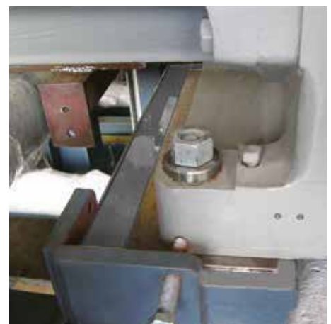
Towing Winch foundation on Chockfast®
