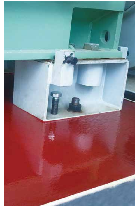
High speed Motor skid mounted on Chockfast®
