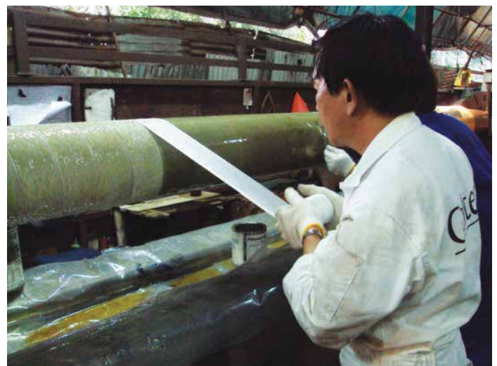
When applied with fiberglass tape, Phillyclad has the ability to withstand hydrostatic pressure
