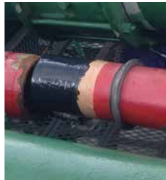
Pipe external coated with Flexane
