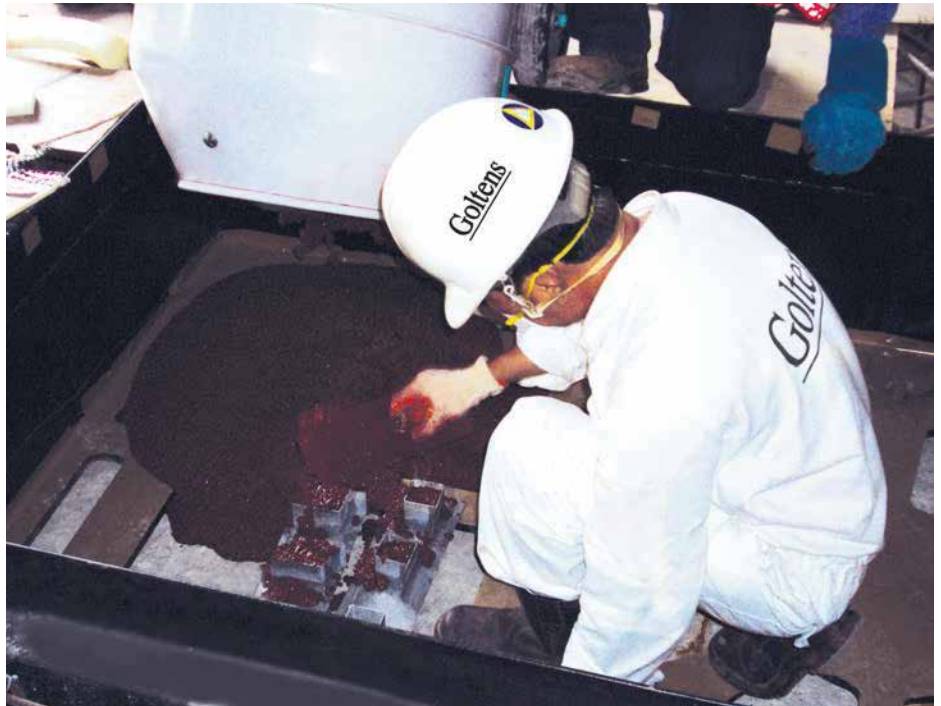
Cube sample taken on Chockfast® for testing
