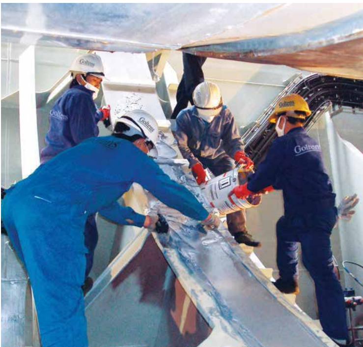
Phillymastic paste application on tank support
