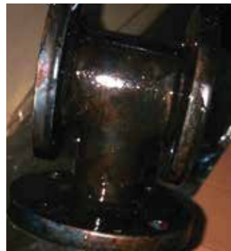
Additional preventive coating for new valve
