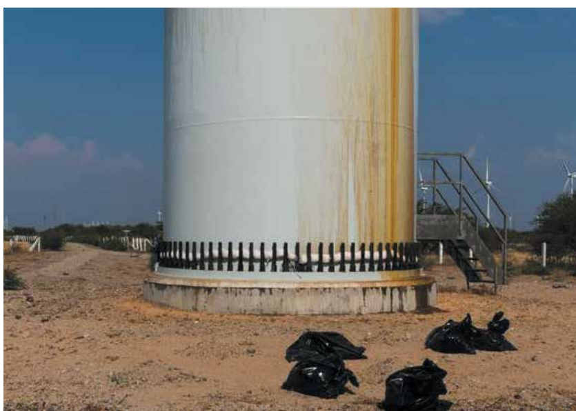
Typical PP absorbent boom failed to absorb lubricant oil
