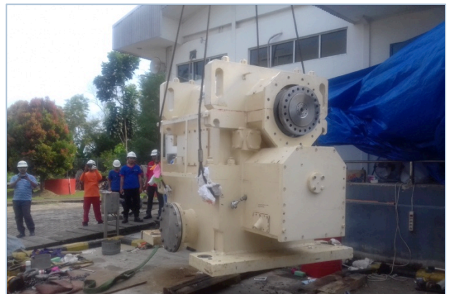
Rigging gear box out of powerhouse to work area
