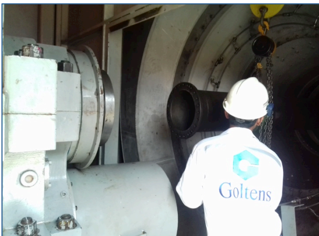
Installation of shaft between gearbox and turbine
