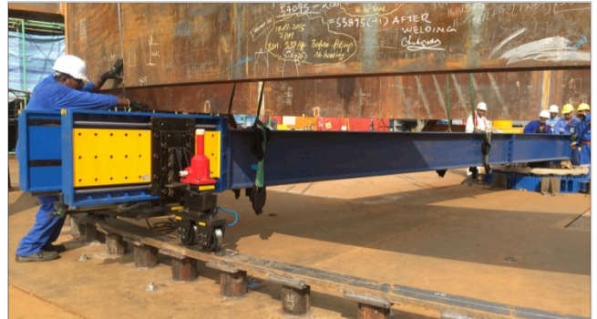
Milling machine installation on running rail
