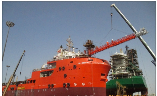
Connecting Flare Boom to King Post
