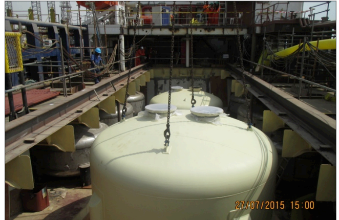
Installation of Acid tanks
