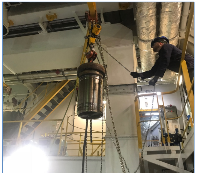
Rigging of liner to calibration/overhaul area
