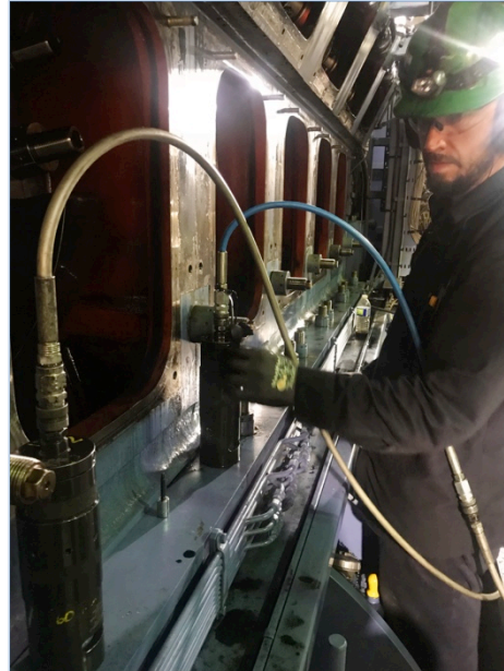
Torque checks of critical fasteners
