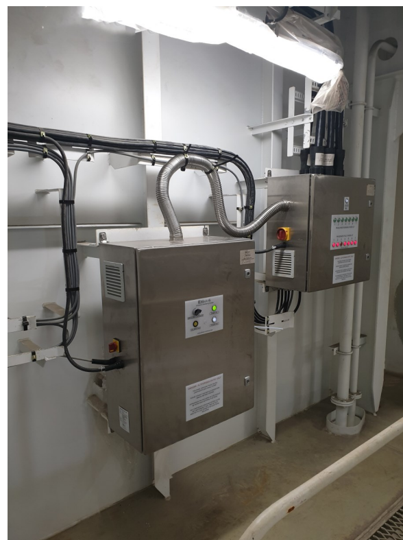
Emsys-iS HLCU variant installed on an LNG Carrier for methane slip and mass emissions reporting
