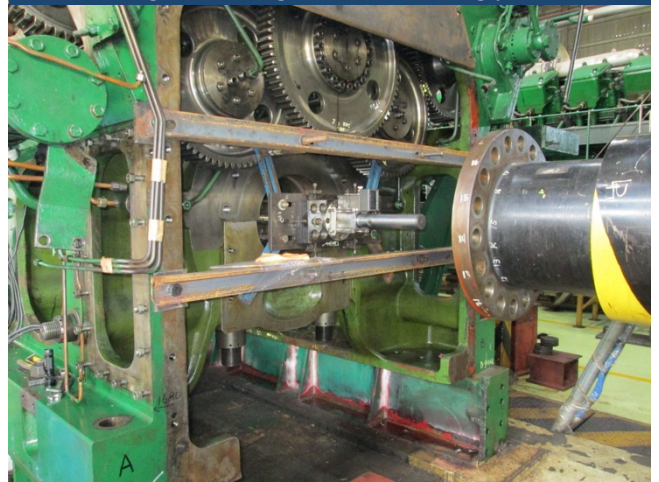
Laser alignment of the engine and generator
