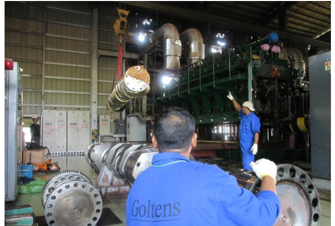
Rigging of the replacement crankshaft
