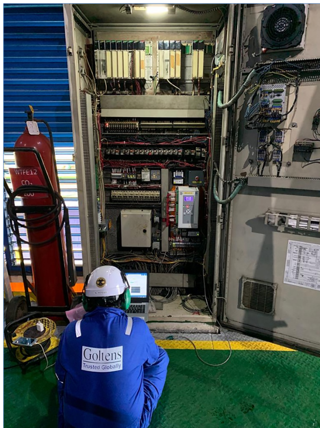
Goltens' controls technician monitoring M5 DG unit during commissioning
