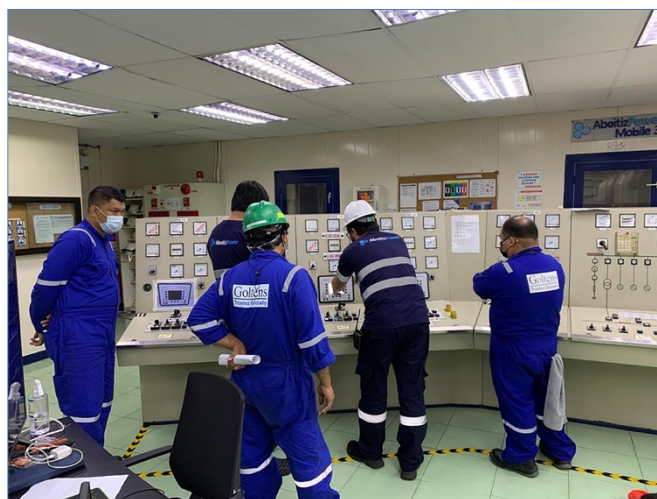
M3 Commissioning of control panel after upgrade with easYgen 3200XT
