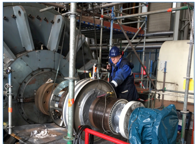
Machining slip ring with single point cutter
