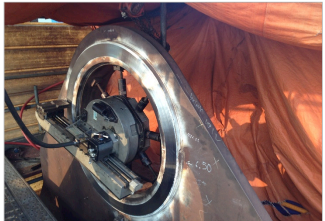
Flange facing of thrust bearing on the base frame
