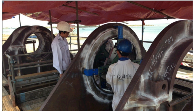
Line boring of the base frame holes
